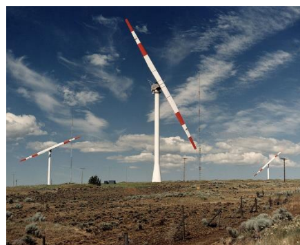
Fig. 2. NASA MMOD-2 wind turbine with a capacity of 7.5 MW in Washington Goodeno Hills, America
